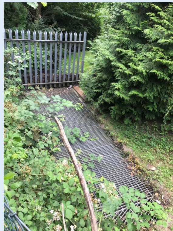
1) Outfall south of carriageway
