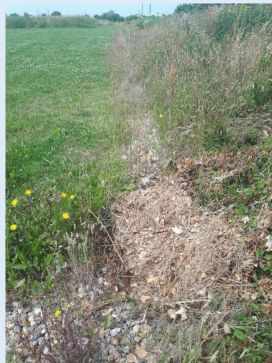
1) View of ground above culvert south of Onshore Order Limit
