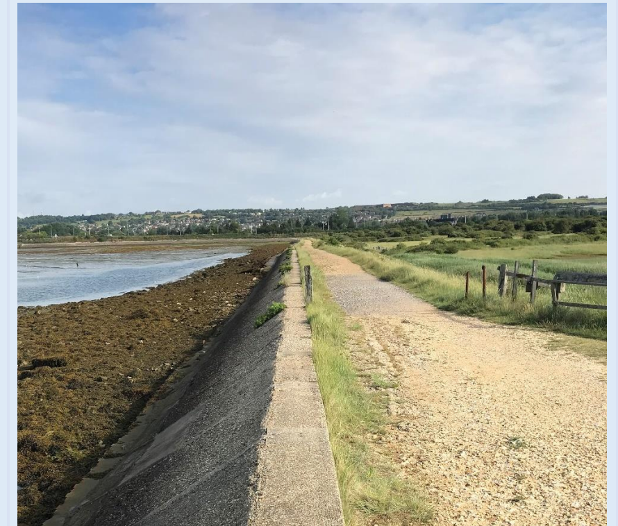
3) Flood Defence prior to outfall into Langstone Harbour
