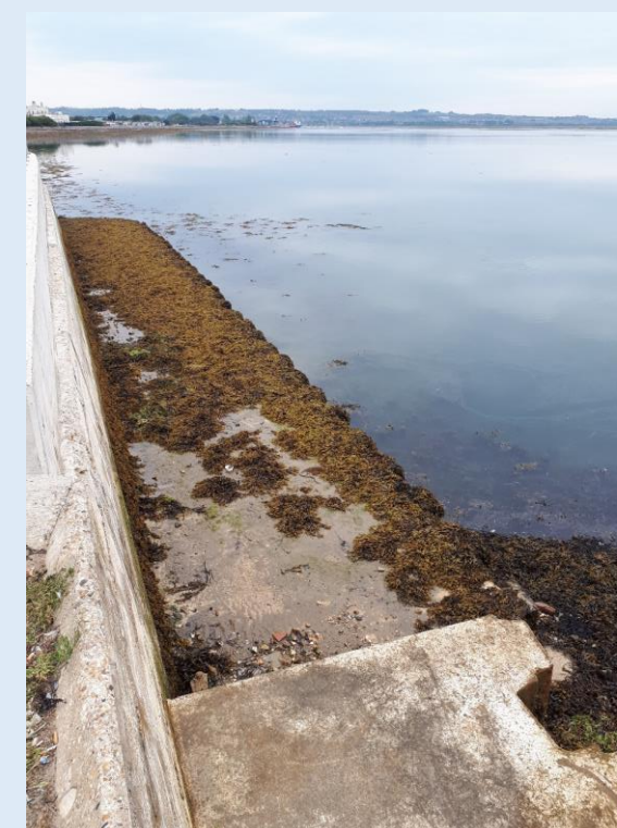
2) Outfall to Langstone Harbour
