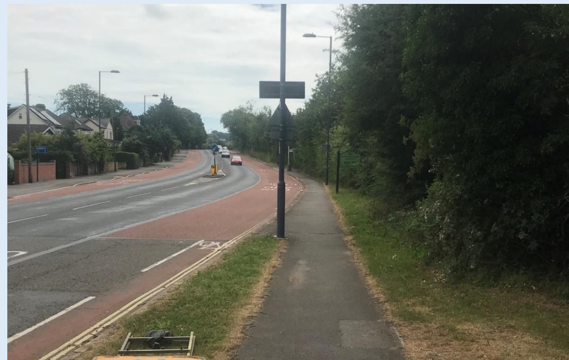
1) View of north looking south along carriageway, where upstream end of watercourse is anticipated.
