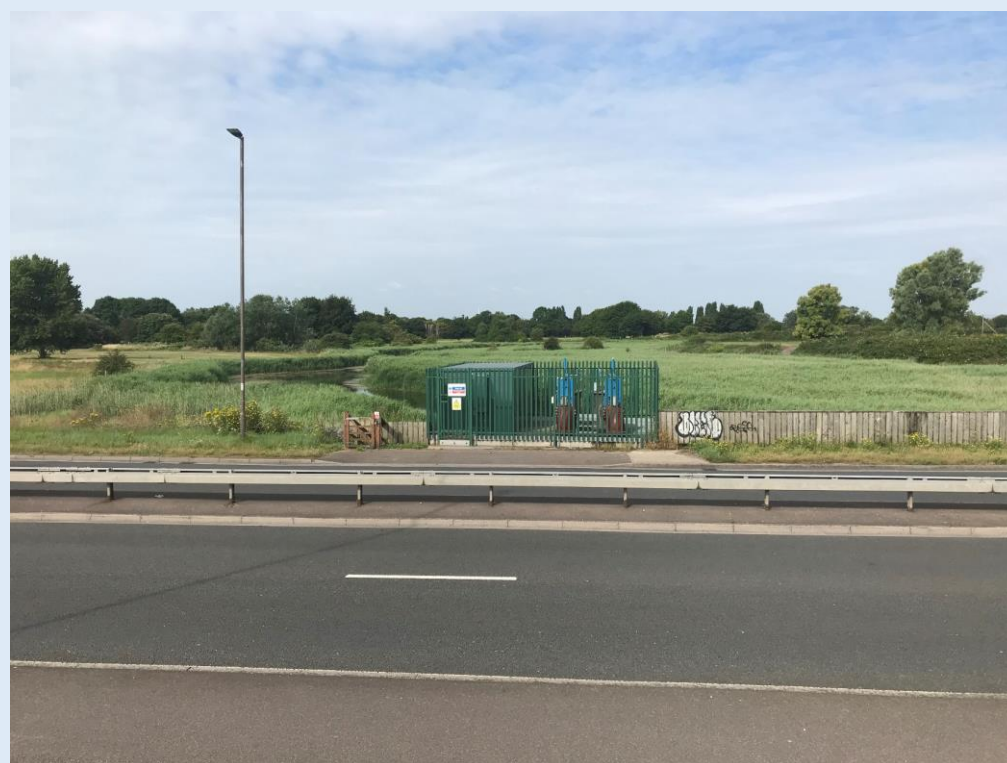
1) Pumping station and carriageway over culvert
