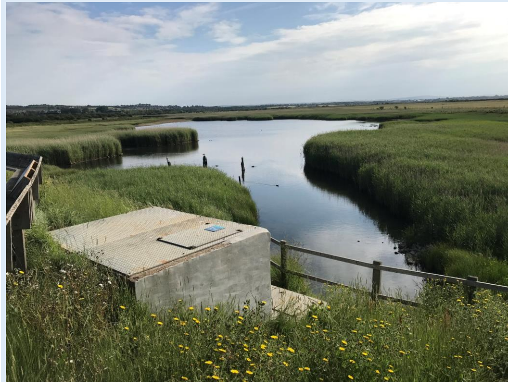
2) Downstream end prior to outfall through flood defence
