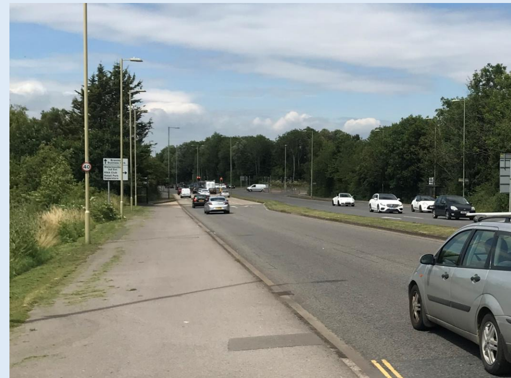
2) View of carriageway above culvert
