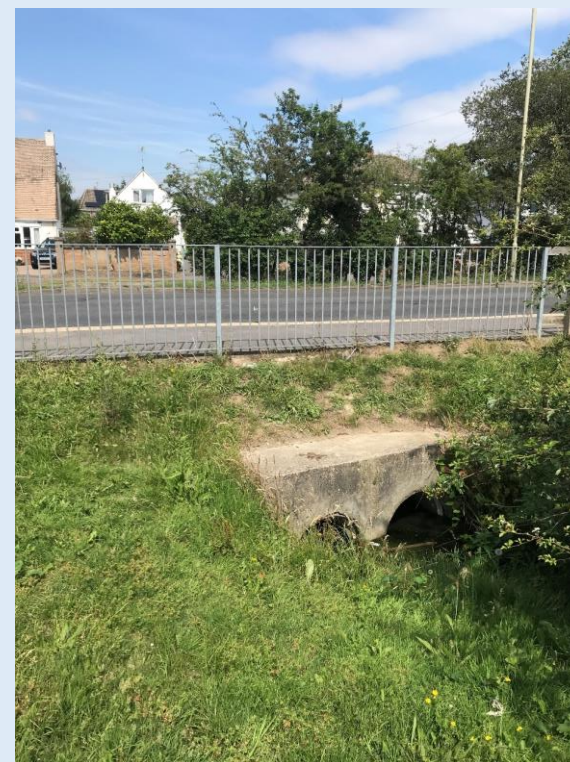
2) View of culvert outfall south of carriageway
