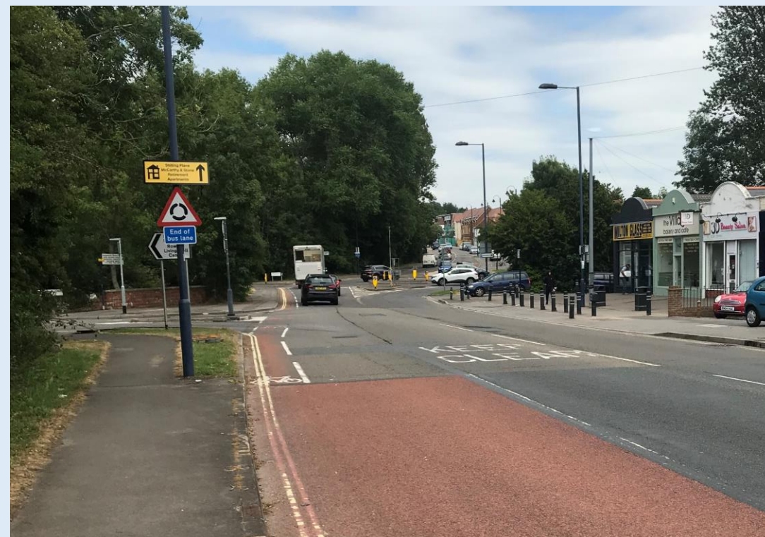
1) Looking north towards carriageway above culvert
